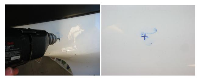
35. Use the hole saw (was provided with the back-up sensor kit in my case) and drill the hole. Make sure to debur the hole, and also redrill the hole again to make sure that enough plastic was removed.
